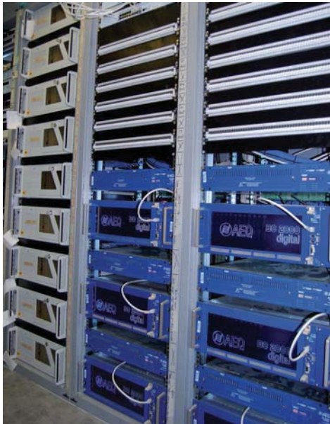
Detail of the Radio Euskadi machine room, where the AEQ-supplied 1024 x 1024 BC2000 Digital matrix stands out.
