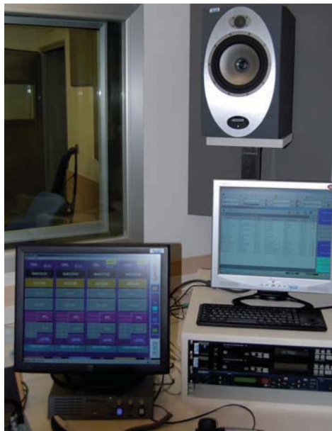
The Basque public radio network keeps a total of 32 ISDN consoles continuously active (these consoles are managed from this Systel 6000)
