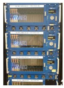
Based upon the BC2000D routing systems and with a total routing capability of over 5000 x 5000 cross-points, the system contains all the necessary elements for interconnection of all the competition venues and the International Broadcasting Centre through long range MADI links over fiber networks. Control of the Commentary System is both local and centralized at the International Broadcast Centre, where all the signals are converging for Distribution to the RHB's.
