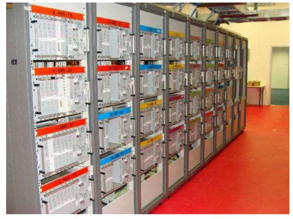
All the interconnections of the 51 stadiums to the IBC were done through 2Mbps E1 links using AEQ RANGER multiplexers, and ISDN lines with the AEQ TLE-02D Portable audiocodec.
